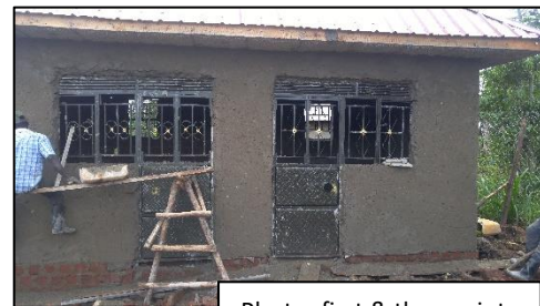
Plaster first & then paint
