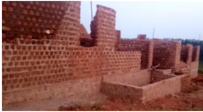
Progress on Paul's house
