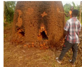
Bricks burned for the 2 rooms
