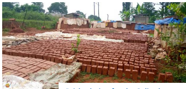
Bricks drying for the Colins house
