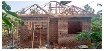
workers are also doing the ceiling boards at the same time. In Uganda the builders do not use sheetrock for a ceiling. Instead they install wire mesh between the rafters and then....well it's hard to explain but see if you can envision this: the builders mix up cement in a bucket, send the bucket up to the worker in the rafters, and he
